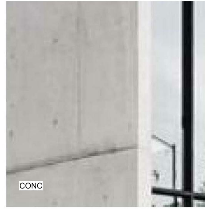
CONC OFF-FORM RAW CONCRETE FINISH
