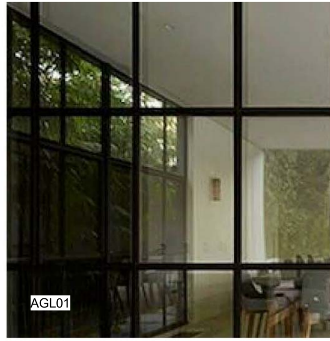
AGL01 CLEAR GLAZING WITH ALUMINIUM DARK CHARCOAL FRAMES
